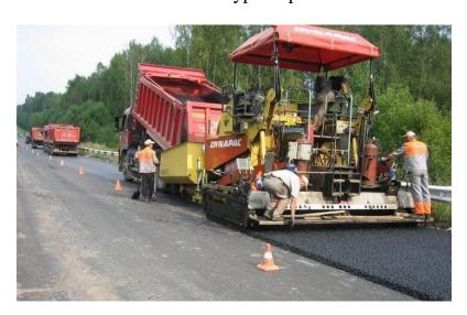
It is recommended to apply up to 5% of bitumen powder out of the total mass of mix while using it for the *production of asphalt mix*.
